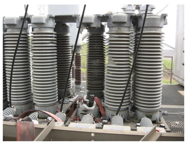
(Figure 9: Single column failure and collateral damage on a porcelain house unit
