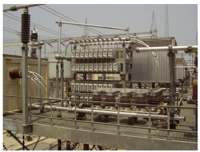
Figure 2: Close up of one Segment of a Series Capacitor Bank Installation. Shown are the MOV units in the front, the triggered gap in the box in the back right, and capacitors to the left of the triggered gap.
