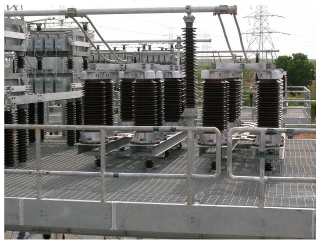
Figure 6: MOV Columns Protecting a Series Capacitor Bank
