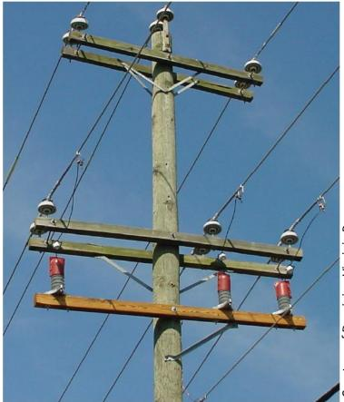
Figure 2 Close-up of Underbuilt Line Arresters
